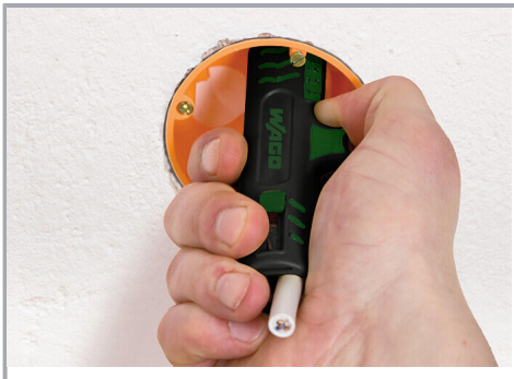
Stripping a cable sheath.
