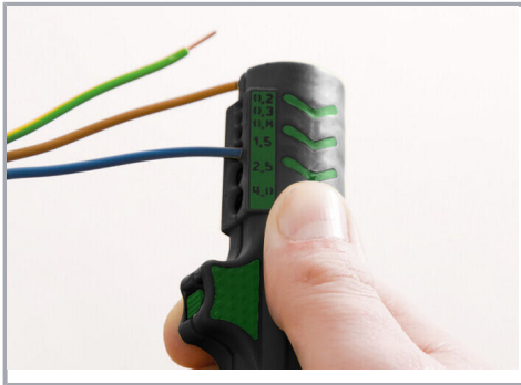
Stripping a wire insulation.
