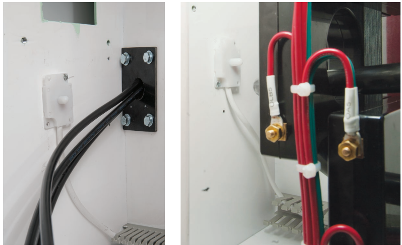
Examples of appropriate point sensor installation.
