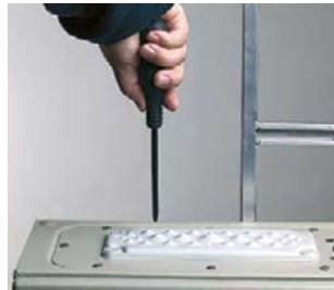
Make a small hole in the membrane.
