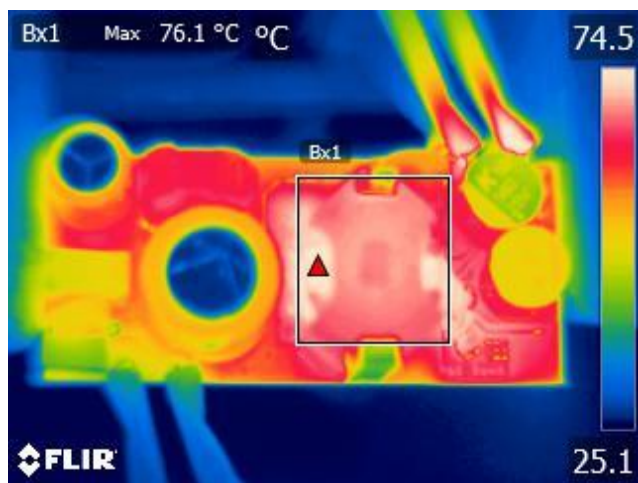
Figure 22 – Ambient = 25.1 °C. Transformer, T2 = 76.1 °C.
