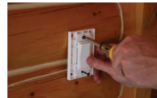
Figure C: Switch Box Mount
