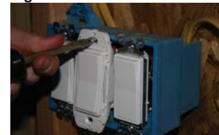
Figure C: Switch Box Mount
