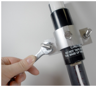
Figure 18. Mast Mount Antenna – Tighten nut on mounting bracket
