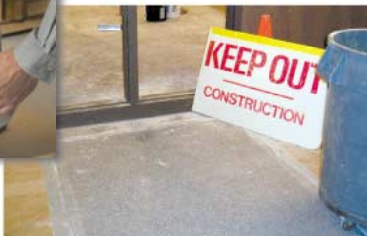
Rubber pressure sensitive adhesive sticks well on contact to metal, plastic, concrete, and other surfaces.
