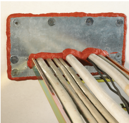
Firestop multiple penetrations: 3M™ FCS-195+ Composite Sheet with 3M™ Fire Barrier Moldable Putty Stix MP+ ( pgs 36-37 )
