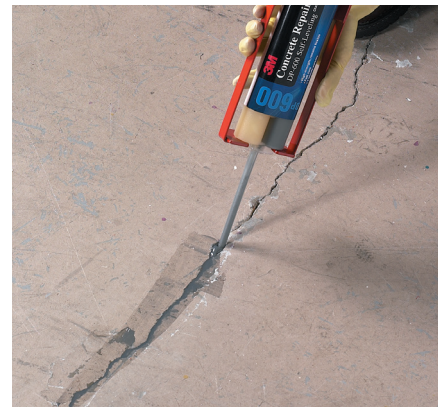
Self-leveling concrete repair: 3M™ Concrete Repair 600 ( pgs 27 )
