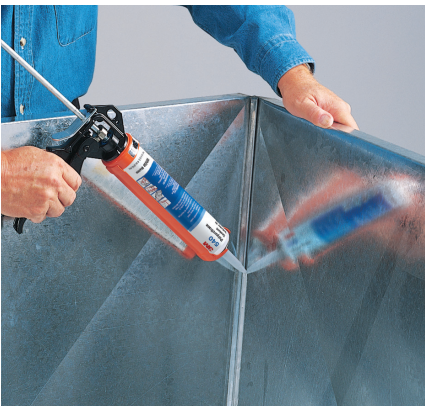
Interior sealing: 3M™ Polyurethane Sealant 540 (pg 30 )
