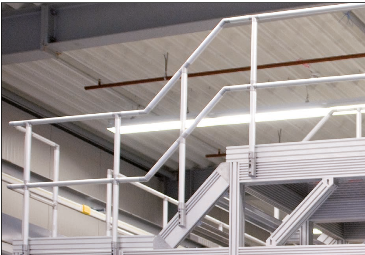
Staircase between two operating platforms.
