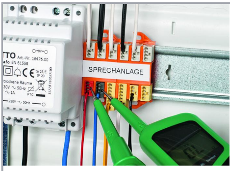
Testing via test port opposite to conductor entry.
