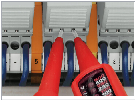
Function testing via touch-proof test slots
